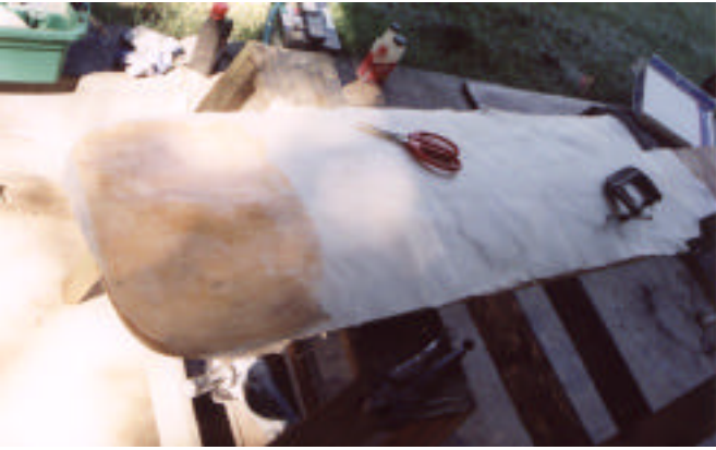
a79. Laminating the exterior with a layer of fiberglass cloth and epoxy.
